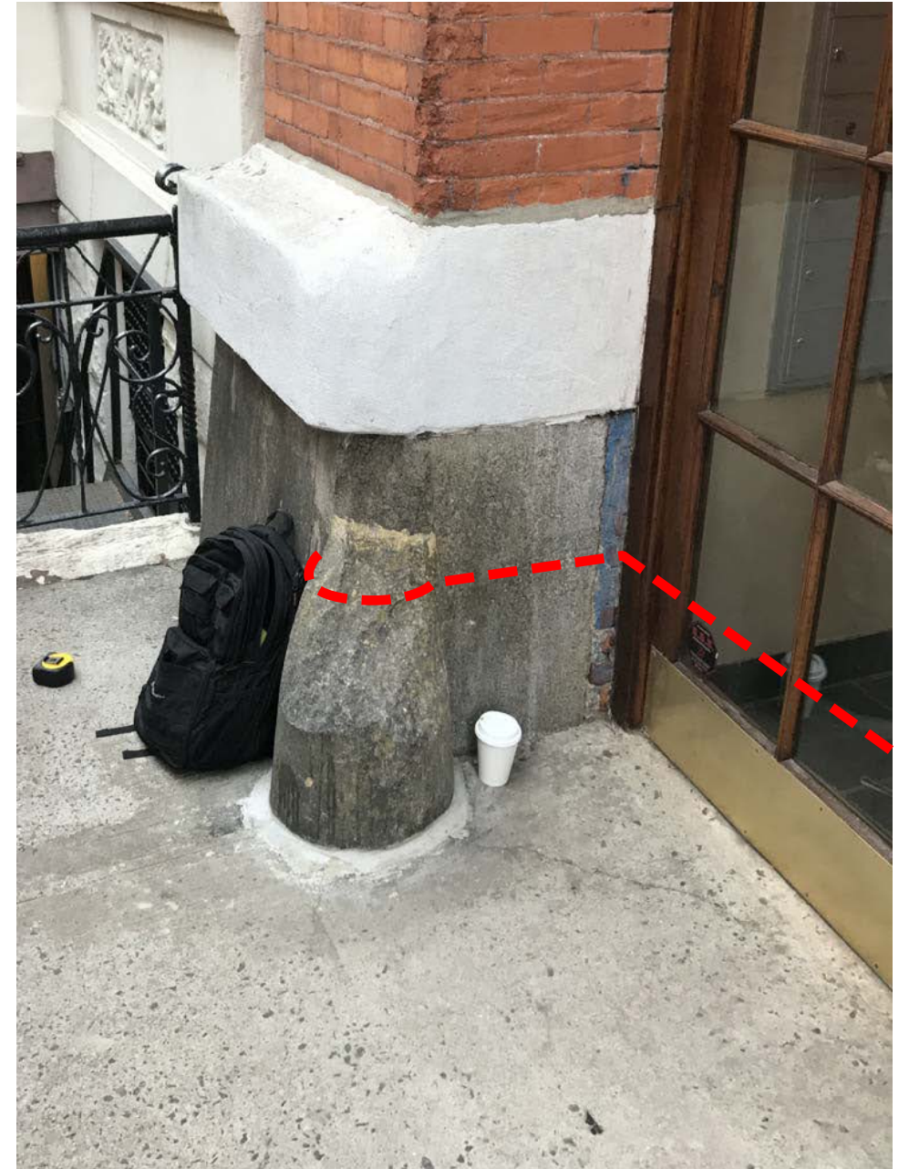
3 EXISTING CONDITION PHOTOGRAPH
