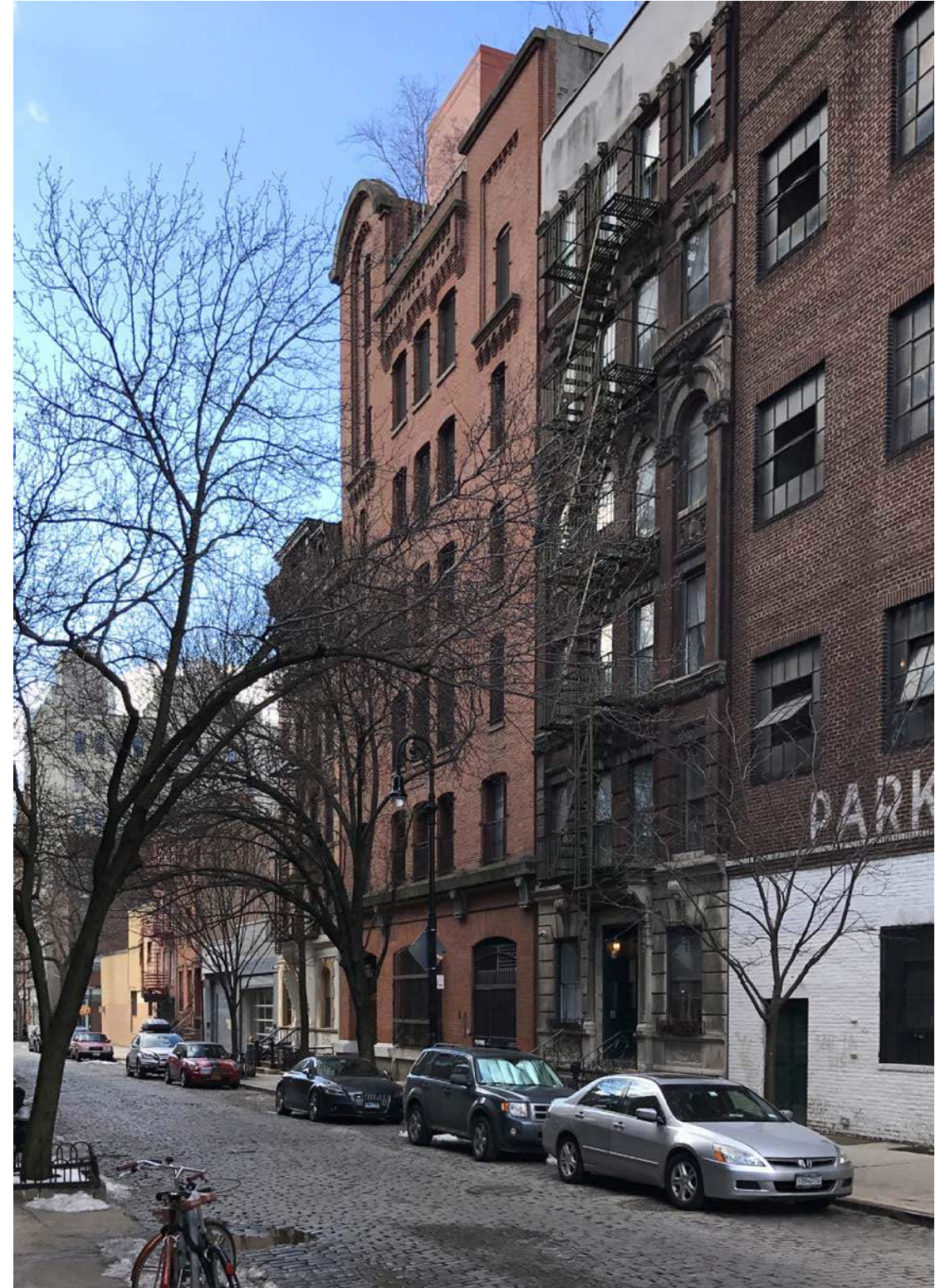
5 EXISTING CONDITION PHOTOGRAPH - FACING WEST
