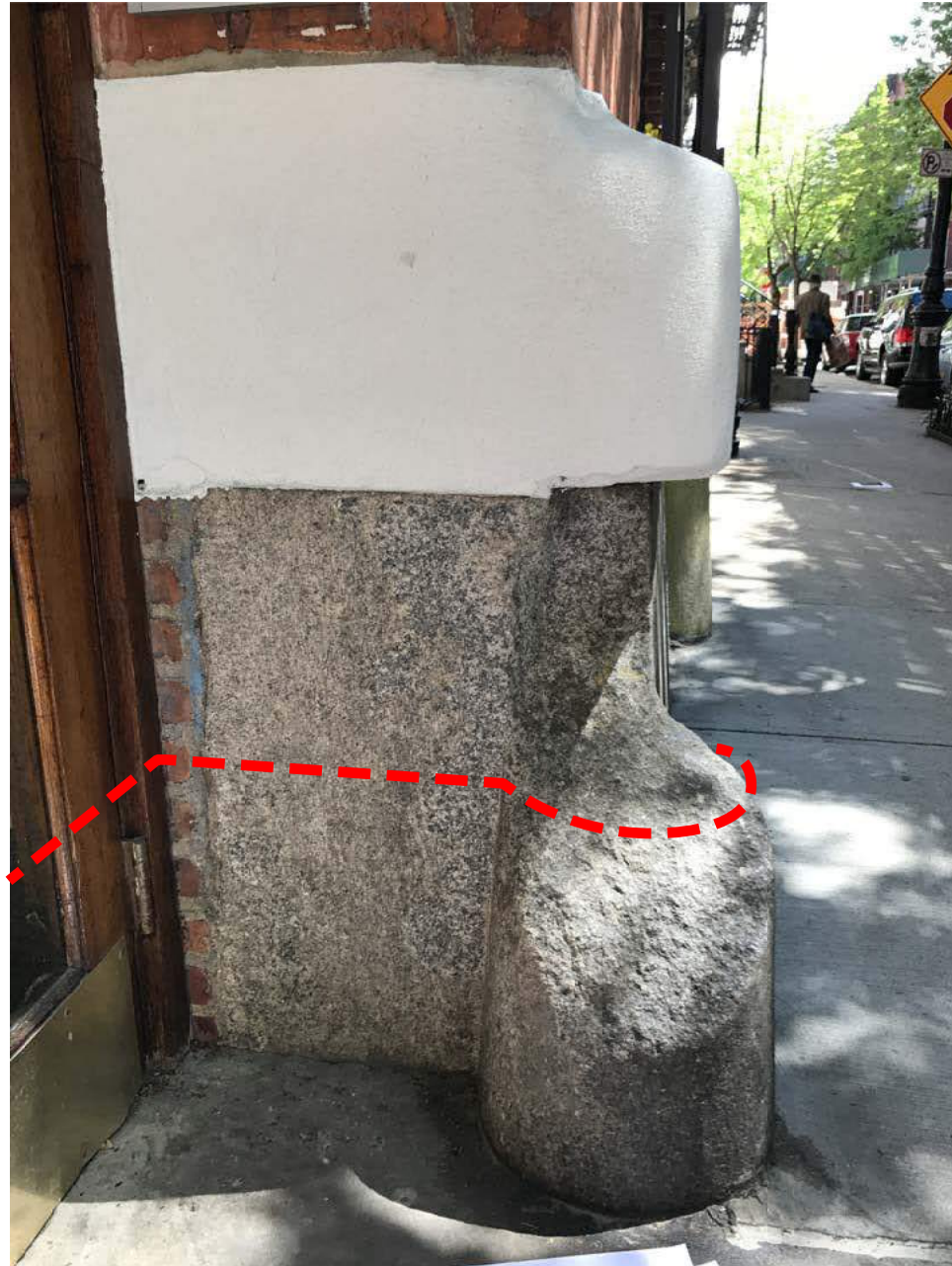
2 EXISTING CONDITION PHOTOGRAPH
