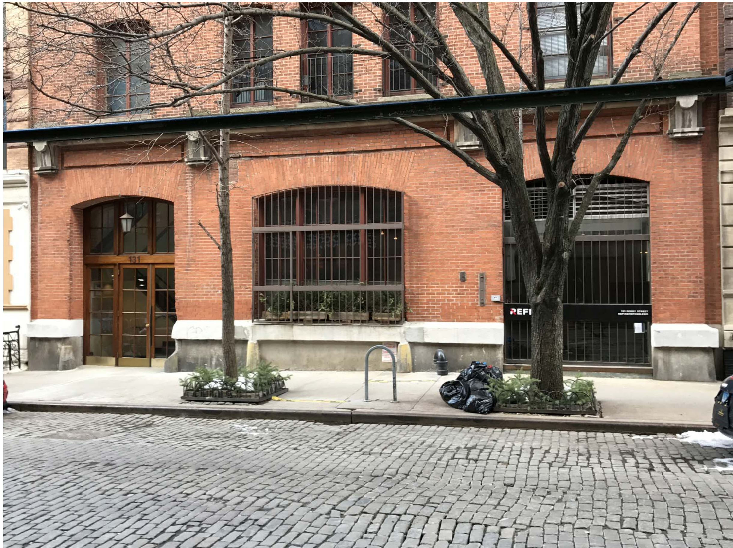
EXISTING CONDITION PHOTOGRAPH - FACING NORTH
