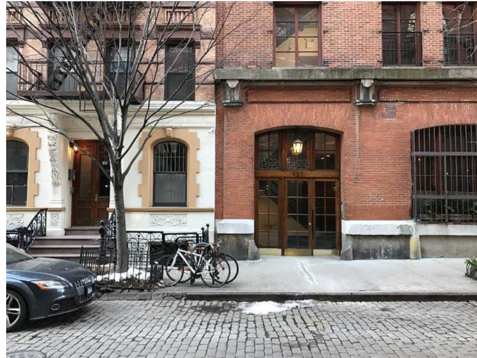
2 EXISTING CONDITION PHOTOGRAPH - FACING NORTH
