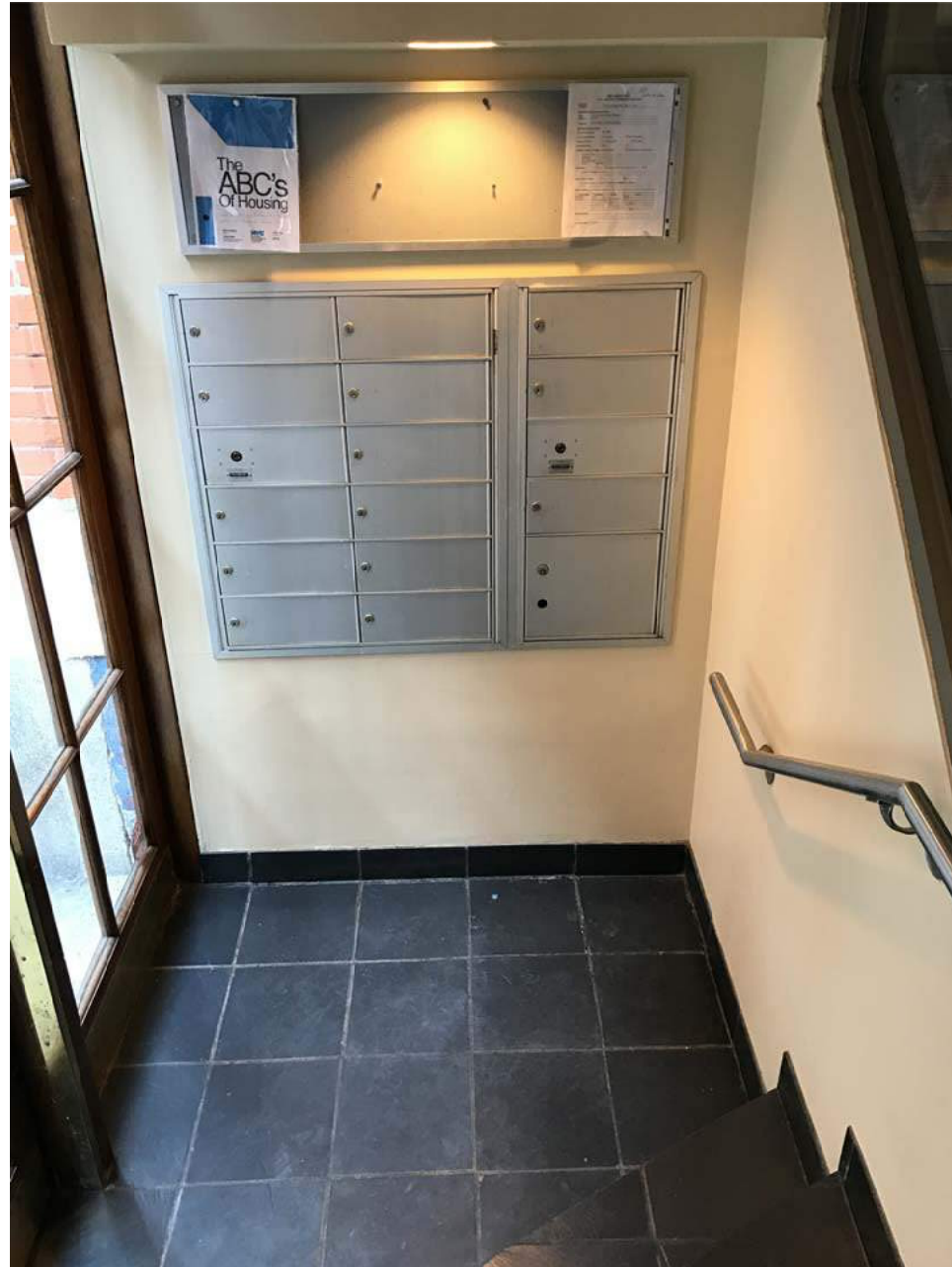
2 EXISTING CONDITION PHOTOGRAPH - VESTIBULE
