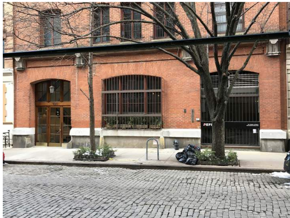
3 EXISTING CONDITION PHOTOGRAPH - FACING NORTH
