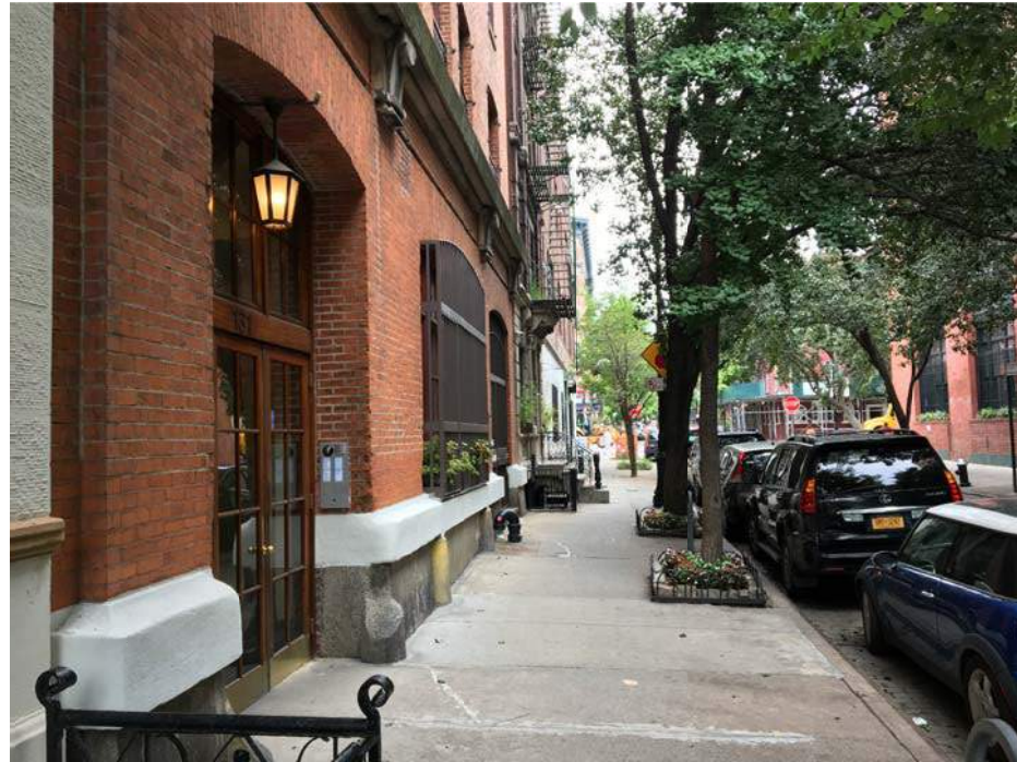
1 EXISTING CONDITION PHOTOGRAPH - FACING EAST
