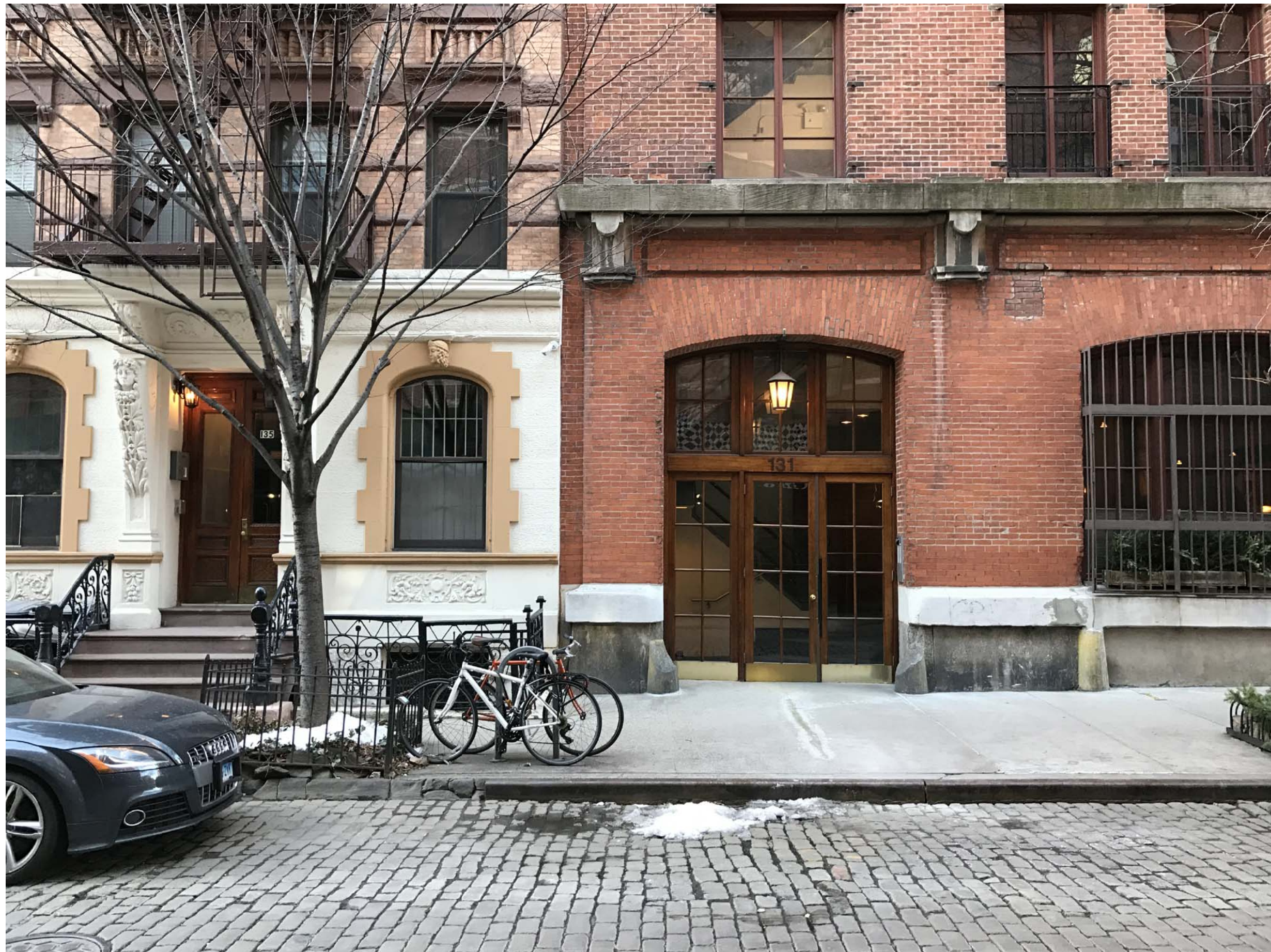
EXISTING CONDITION PHOTOGRAPH - FACING NORTH
