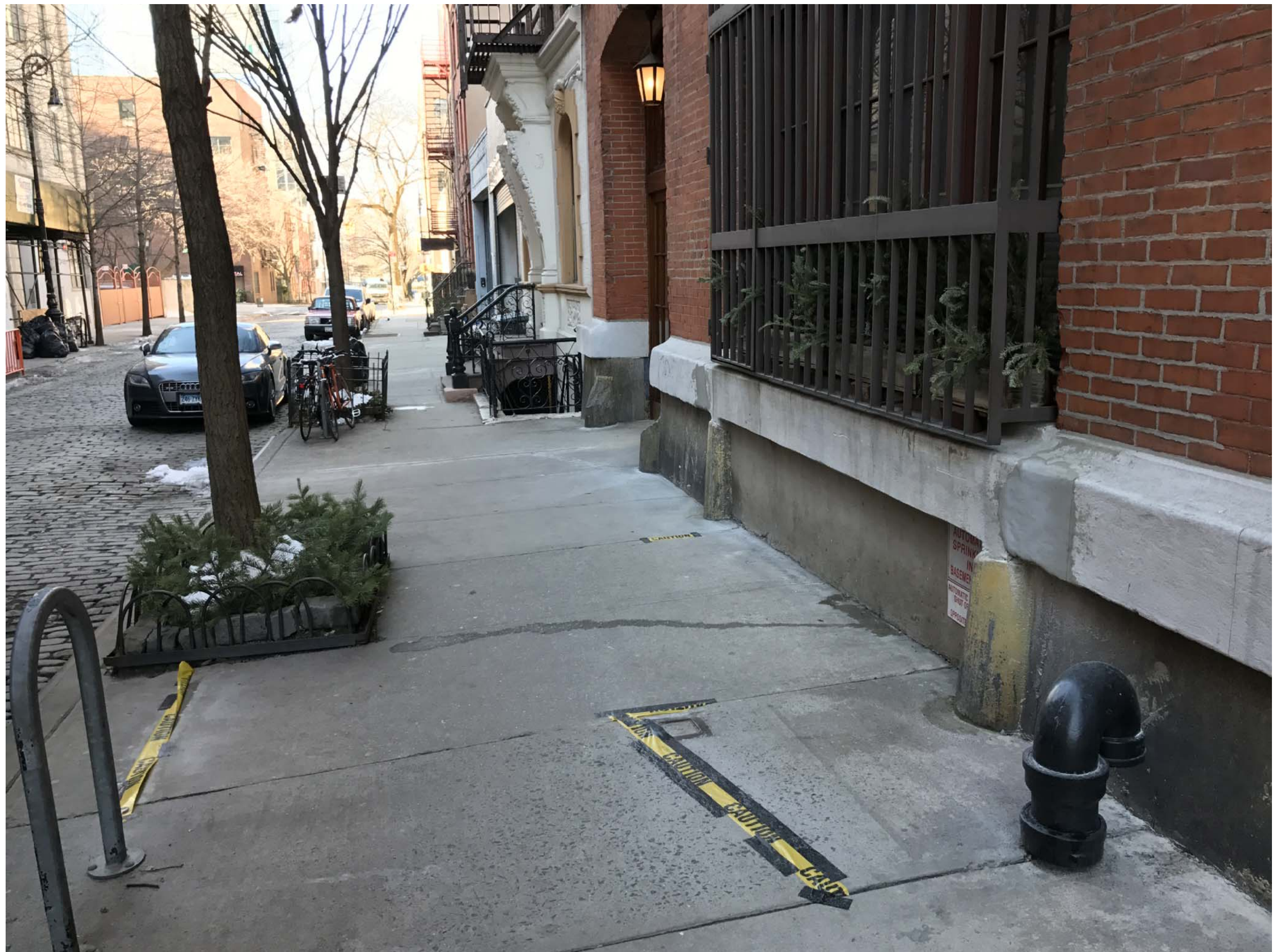
EXISTING CONDITION PHOTOGRAPH - FACING WEST
