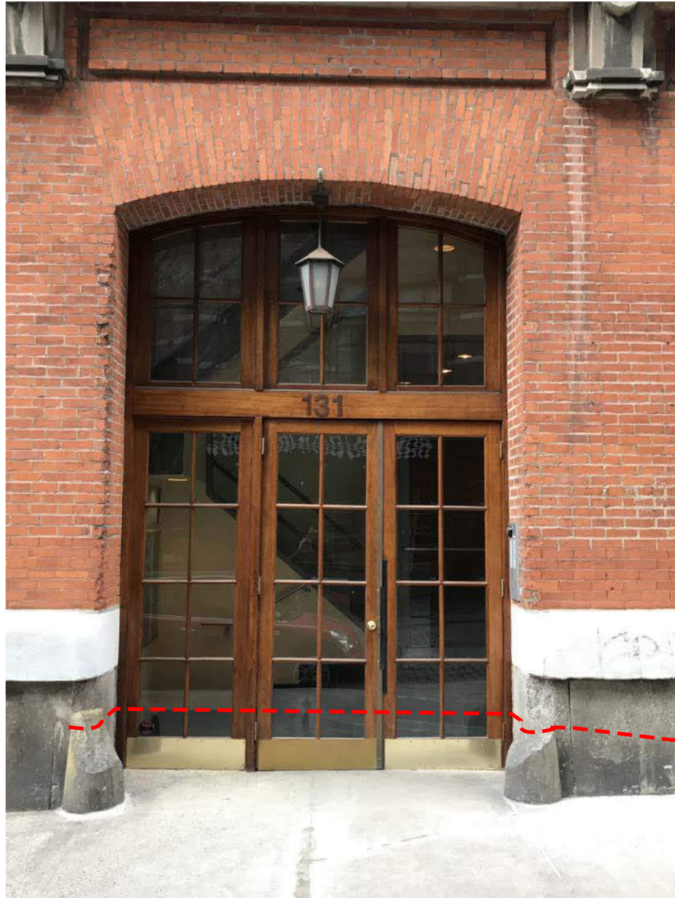
1 EXISTING CONDITION PHOTOGRAPH
