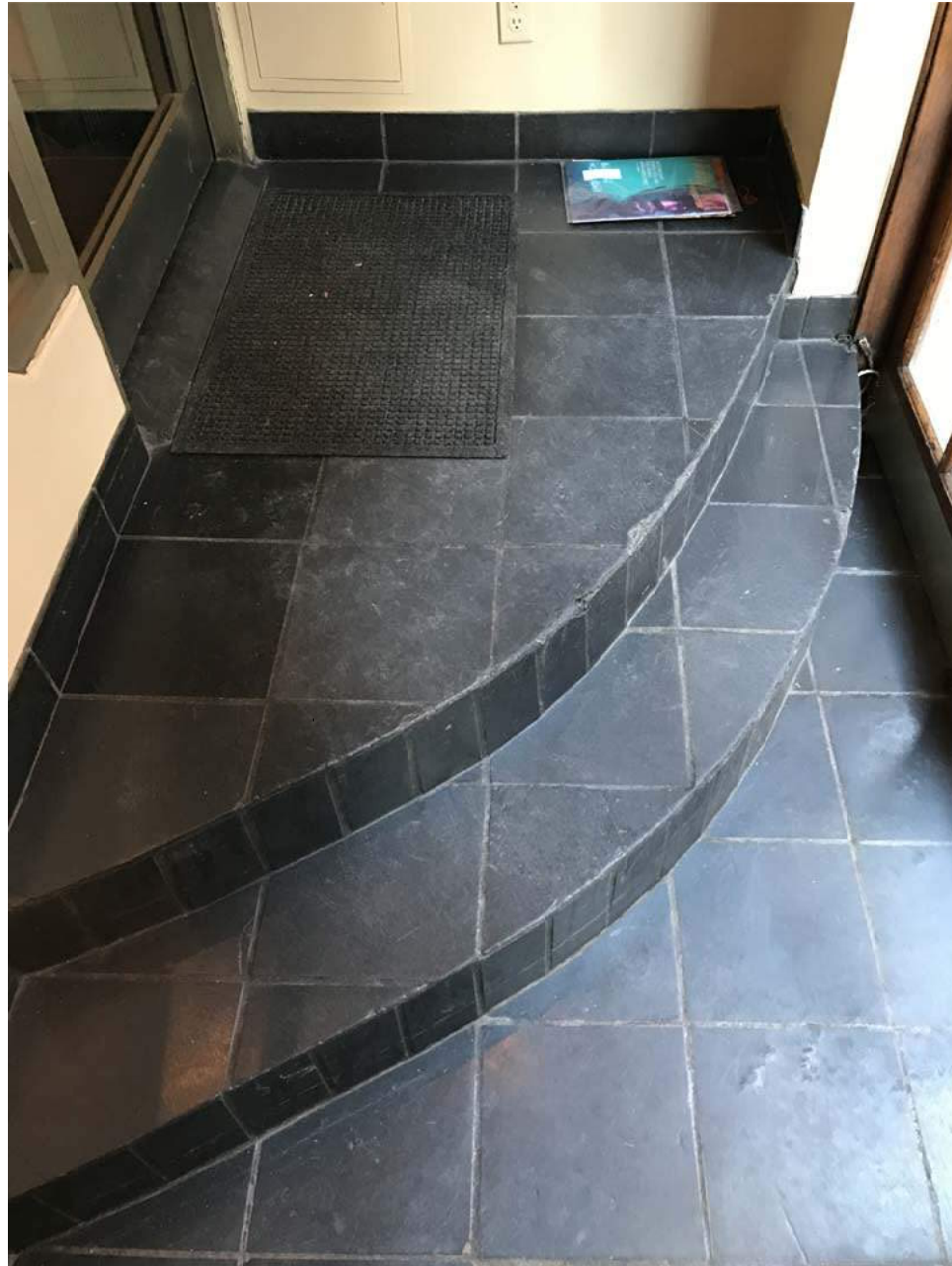
1 EXISTING CONDITION PHOTOGRAPH-VESTIBULE
